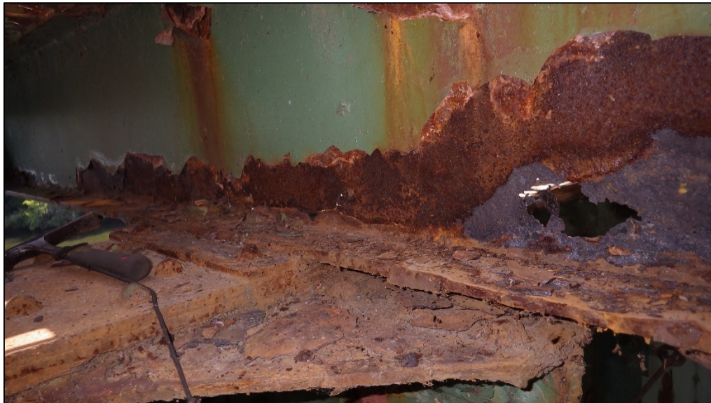
Floor Joists on Approach Spans
