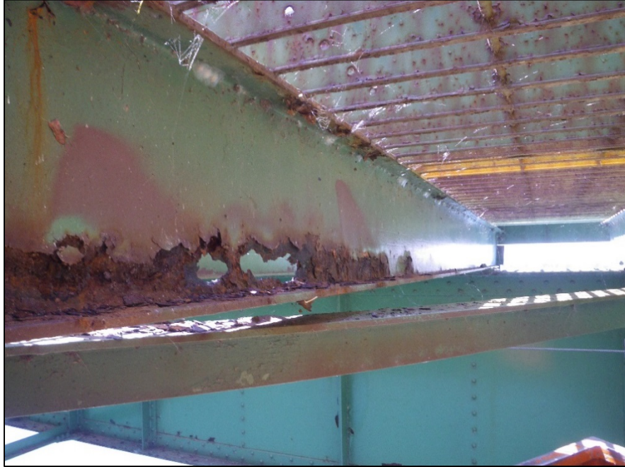
Transverse Floor Joists on Girder Spans
