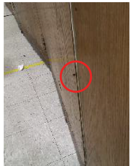
Figure 1 – Protruding Nail
