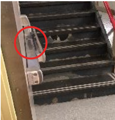
Figure 3 – Thick Layer of Renovation Dust, as Illustrated by the Fingerprint
