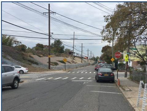
**Image 1** (facing north): Damaged “Stop” pavement marking on the southern leg of Montauk Street
