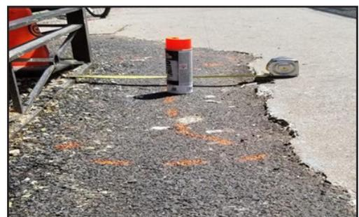
**Figure 5.** 1–2" depression causing a trip hazard on the sidewalk.
