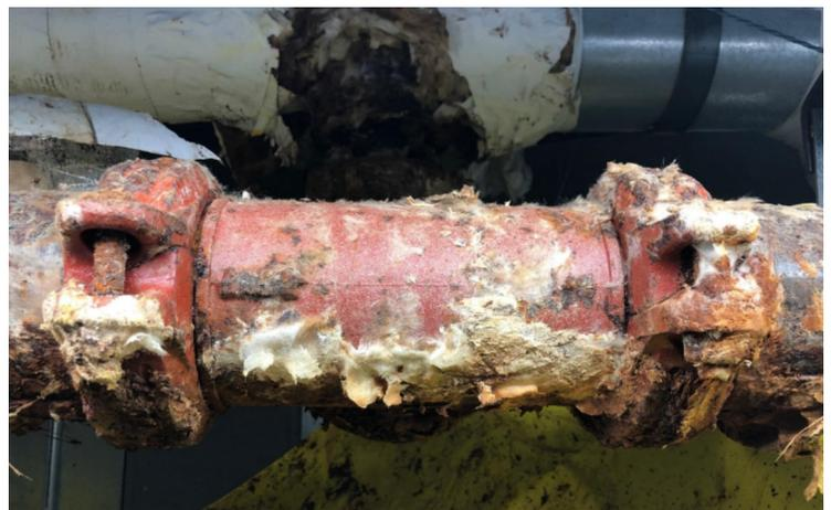
**Picture 3 – Rusted pipe joint at JSBS building**
