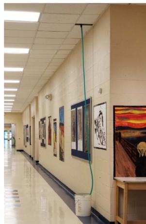
**Picture 2 – Hose and bucket to catch leaks in JSBS hallway**
