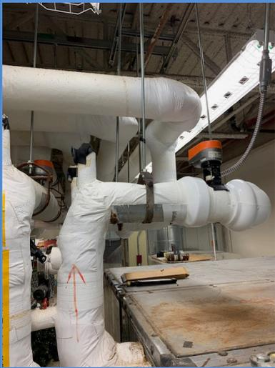
Repairs made to pipes adjacent to air handler AHU #13
