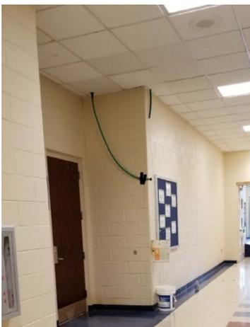
**Picture 1 – Hose and bucket to catch leaks in JSBS hallway**
