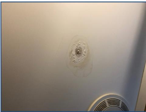
**Figure 2:** Water damage/possible mold.
