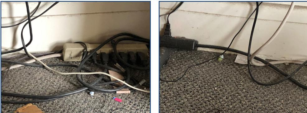
**Figure 1:** Loaded power strip plugged (or “daisy-chained”) into another loaded power strip.
